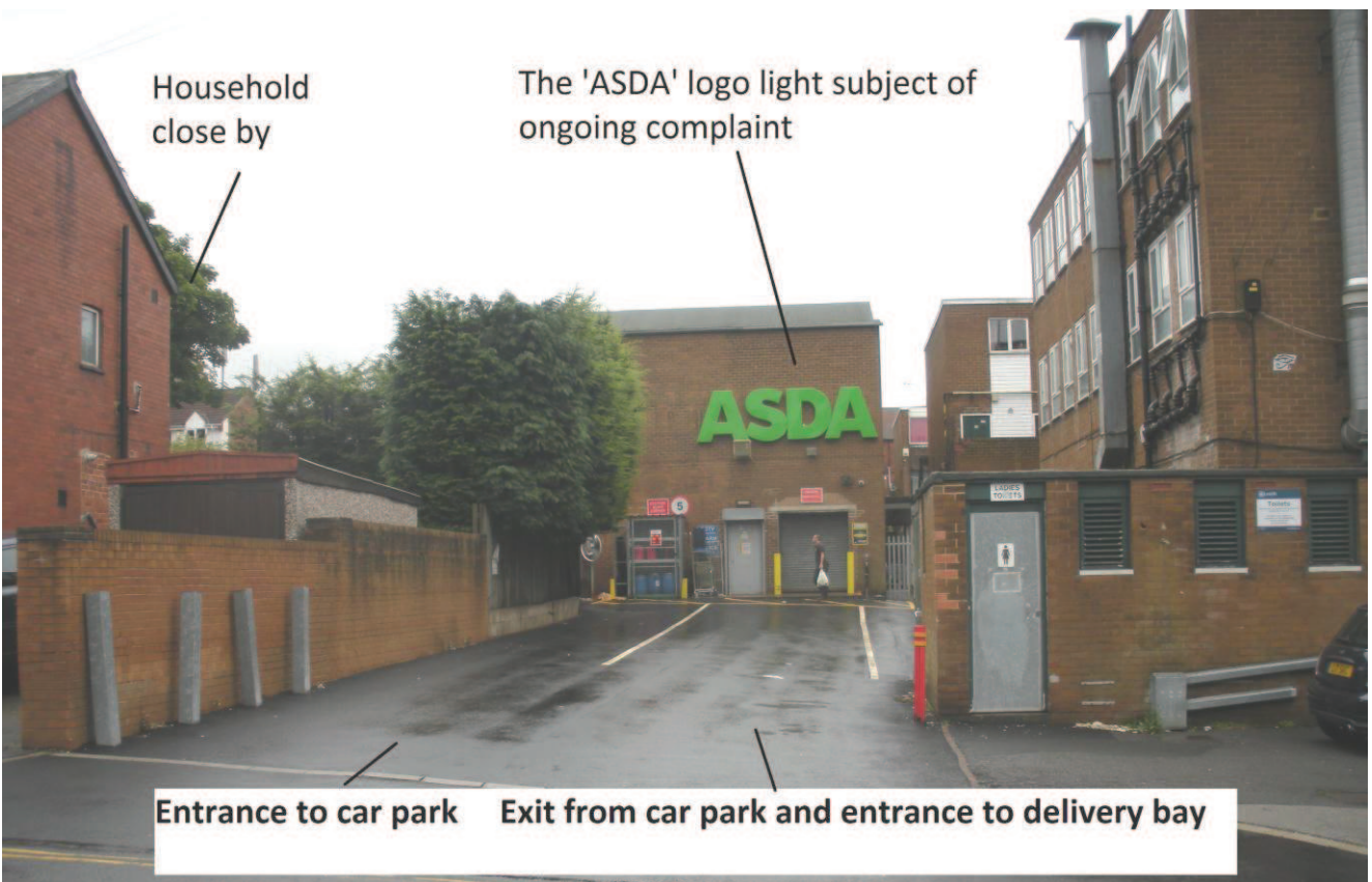
4. Entrance to rear car park and delivery area.
